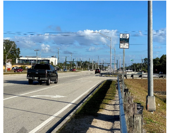
Limited access bus stop on Collier Boulevard
